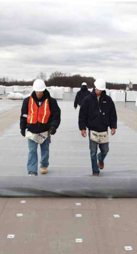
In northern climates, the solar thermal benefits of black EPDM helps to reduce heating costs, which are typically 3-5 times greater than air-conditioning costs. Reflective white EPDM helps to reduce cooling costs in southern climates. The cross-linked nature of EPDM can handle the heat of southern climates.
